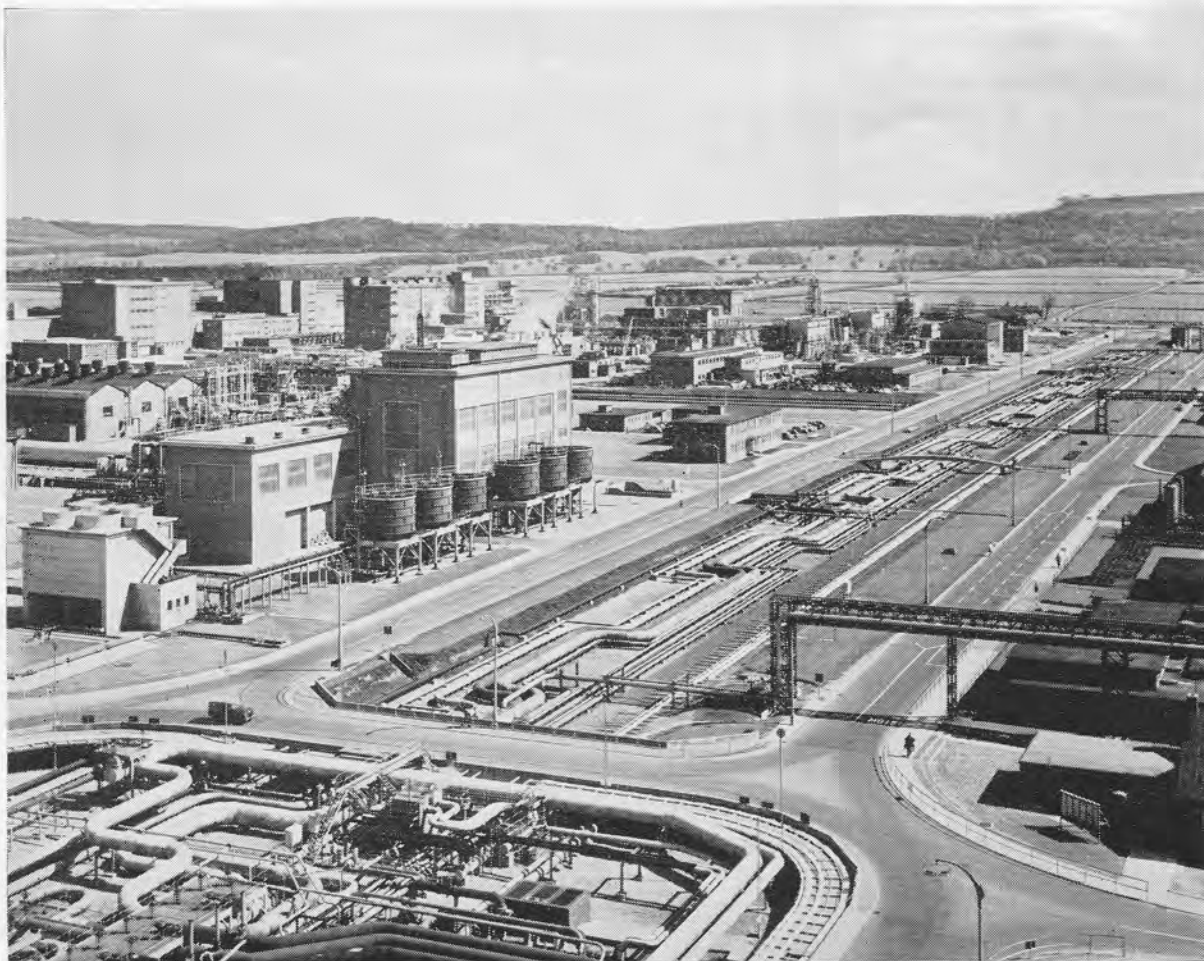
The Wilton factory of I.C.I. on which is situated the plant making 'Butakon'.
